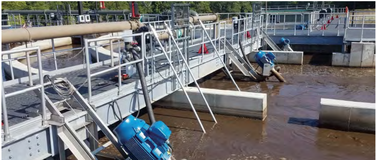
Figure 5: Aeration Industries Triton Aerators
