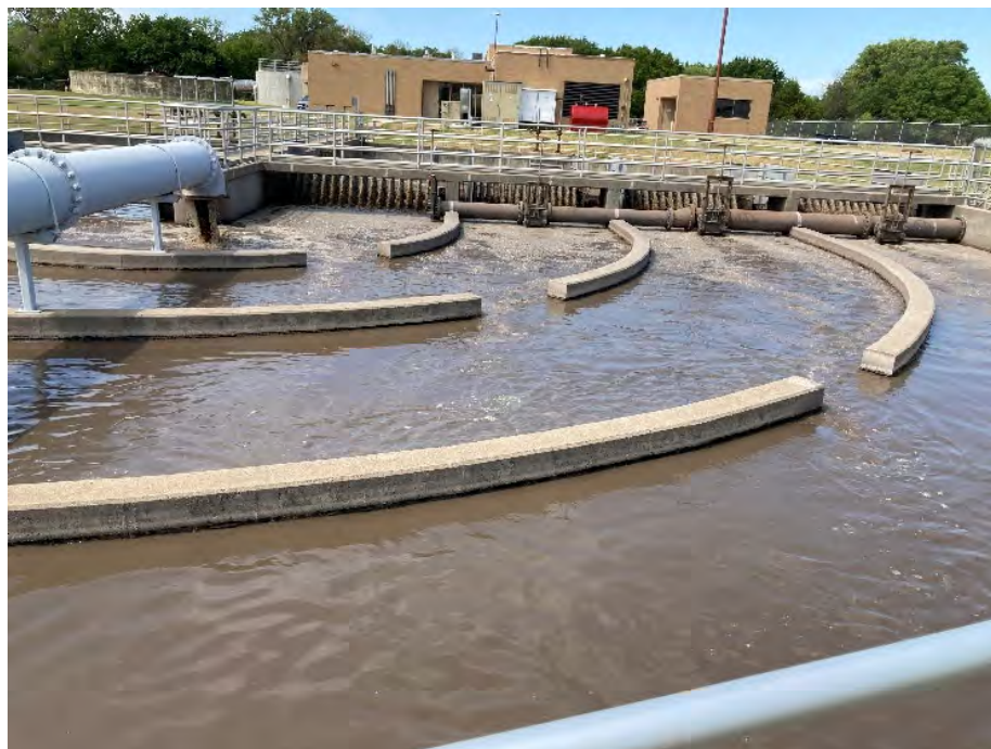
Figure 1A: Orbal Oxidation Ditch with Disc Aerators
