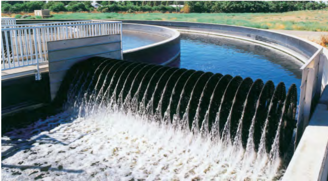
Figure 4: Evoqua OX™ Disc Aerators
