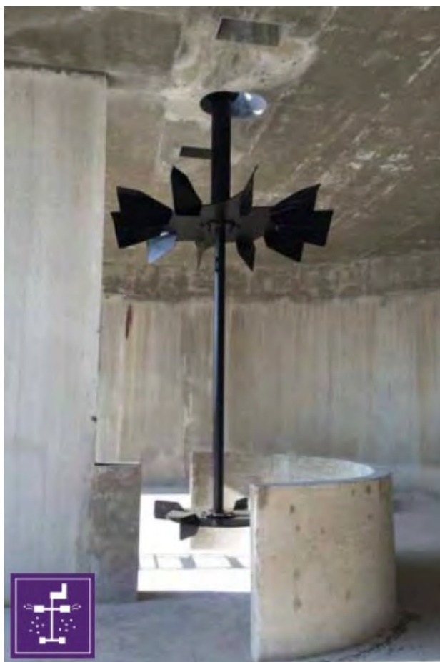
Figure 6: Ovivo Carousel Oxidation Ditch Aeration Equipment
